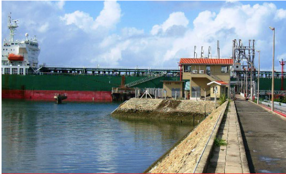
Figure 5: New Kipevu Oil Jetty, Mombasa.
