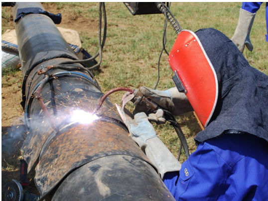
Figure 6: KPC Pipeline Welding and Pumps Maintenance Service
